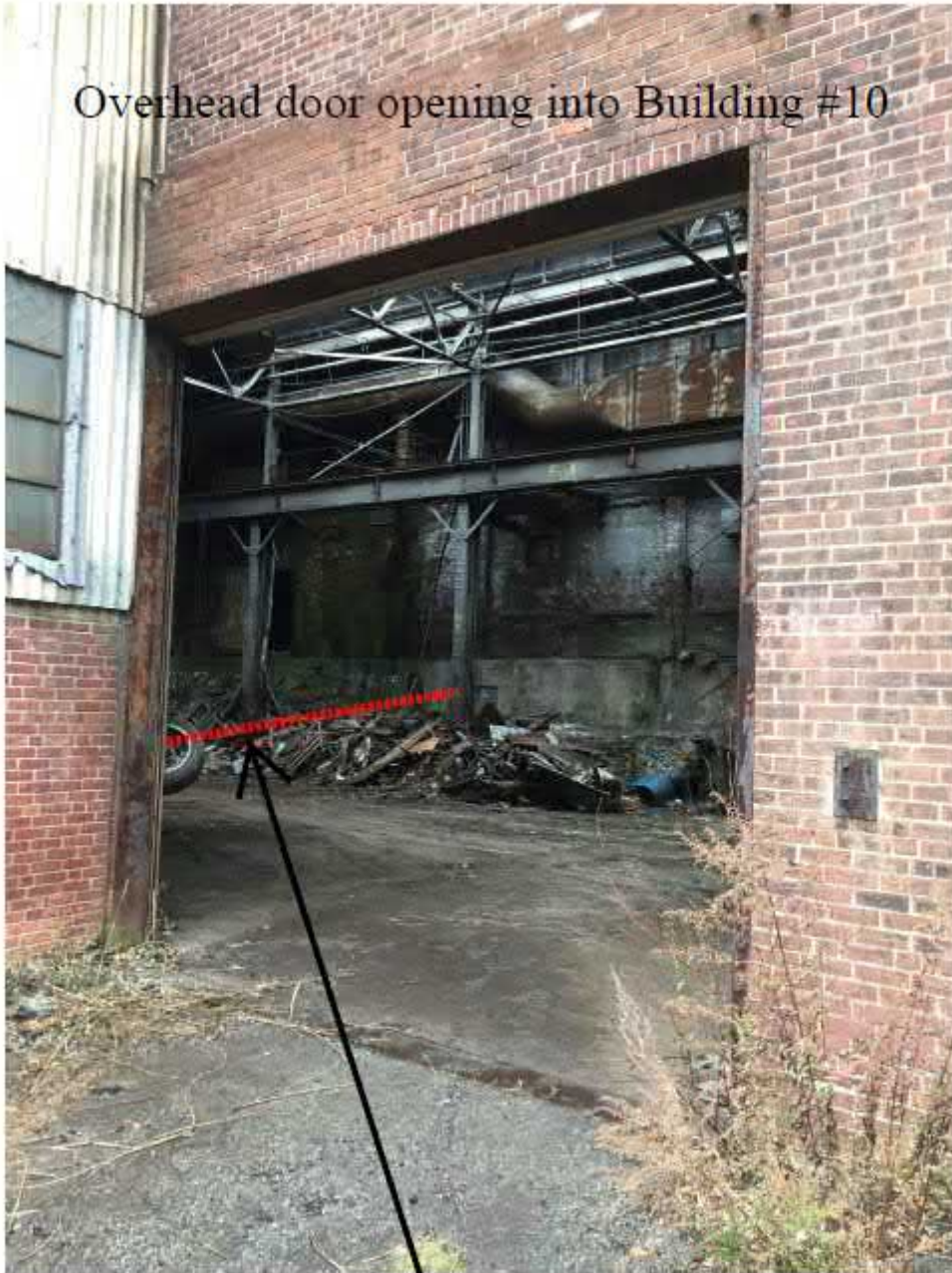
Boundary of initial cleaning for excavator removal
