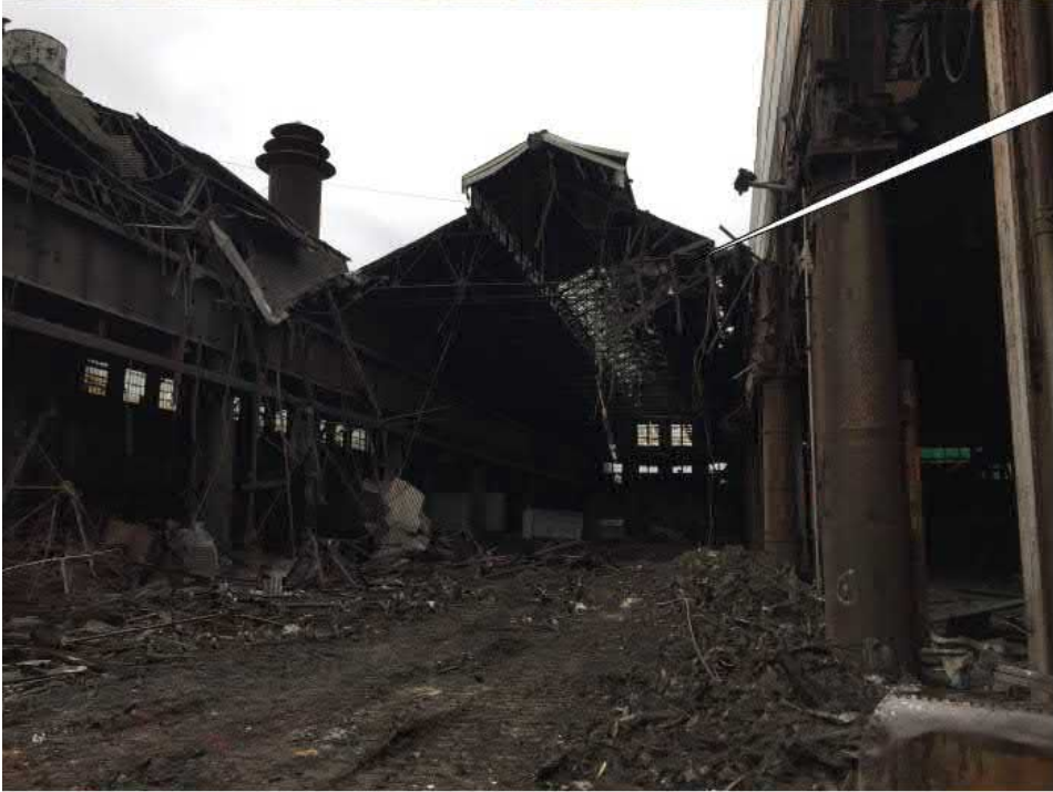
Extent of Demolition
