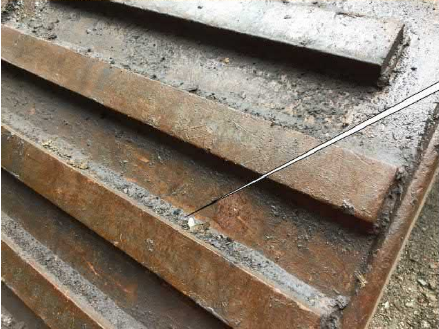
Debris on Tracks
